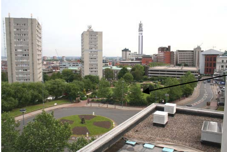
Plate 2.2. View towards northeast from roof of Hall 3 of the ICC with section of roof to be greened in extreme foreground.
