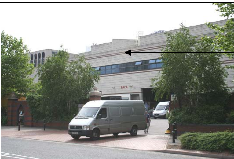
Plate 2.3 View from Cambridge Street of Hall 3.
