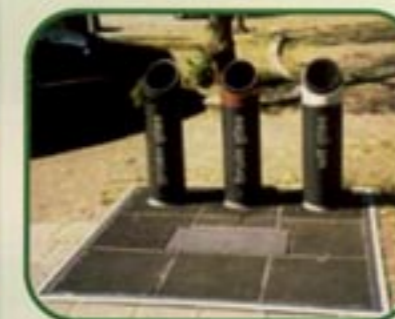
Underground glass recycling container (Dordrecht)
